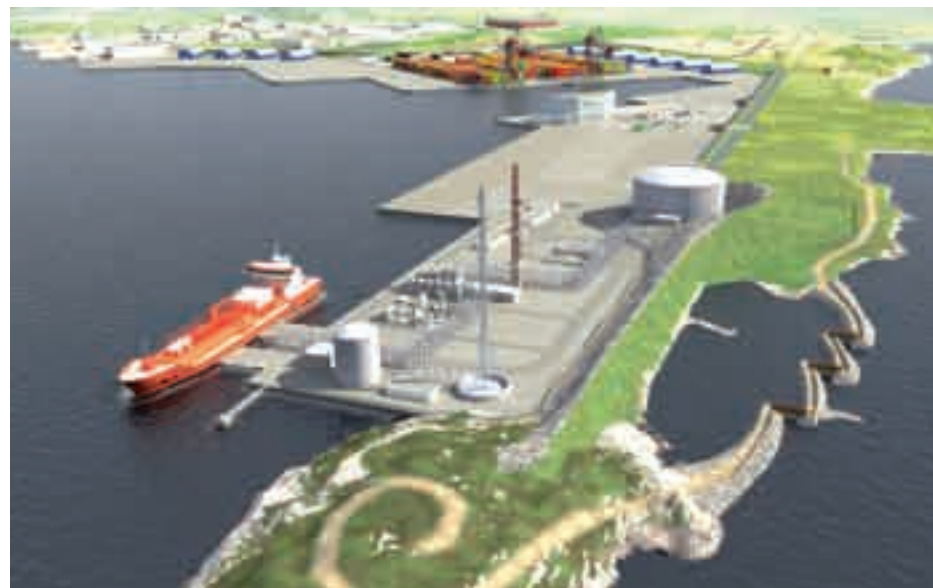
Nordic LNG's 300,000 t/y gas-liquefaction plant comes on stream in 2010
