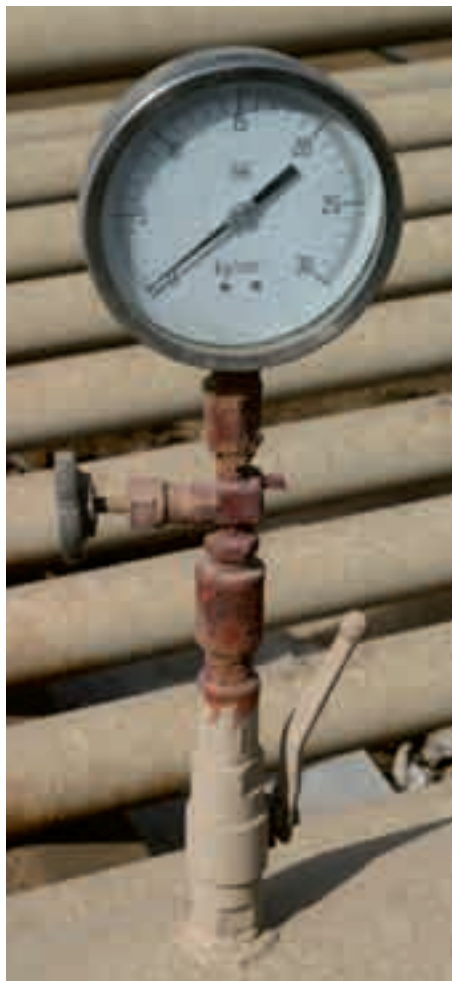
Iraq's gas infrastructure is barely developed, but just $5bn is needed to develop Akkas and Mansuriyah
